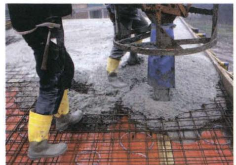
In-situ reinforced concrete being poured
